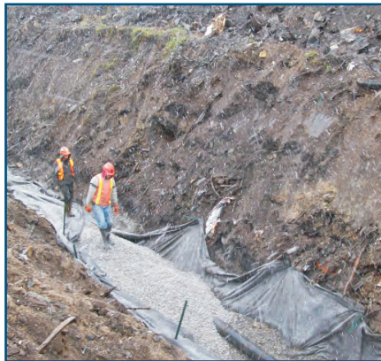
Construction of leachate collection trenches and retention pond
