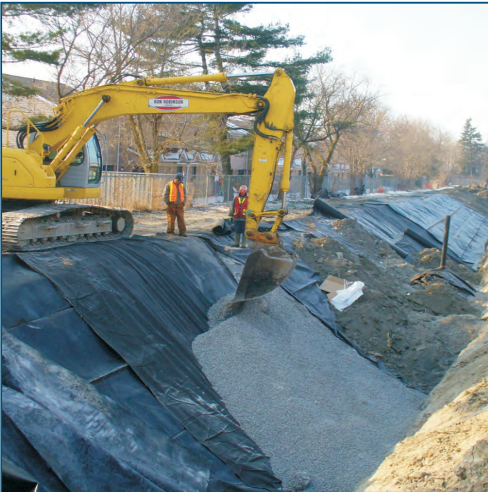
Work on the gas venting system.
