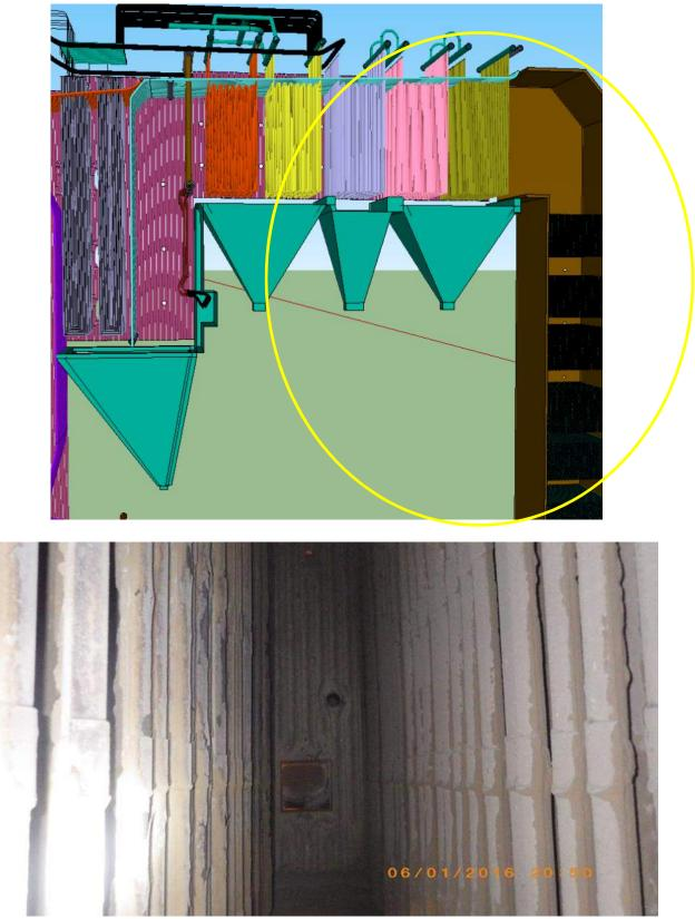
Photo 14 - View Between Superheater Sections - Fouling Typical
