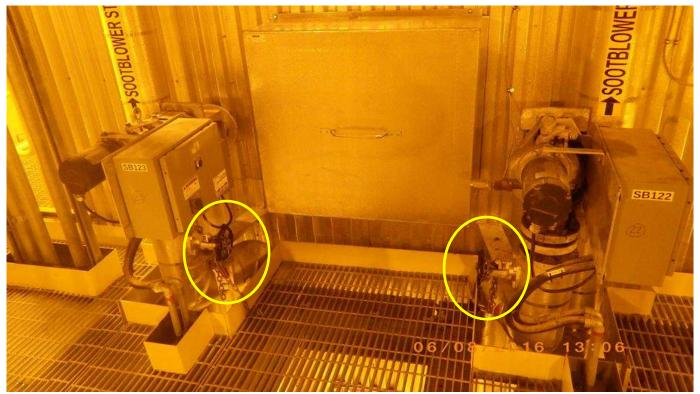
Photo 18 - Economizer Sootblowers 122 and 123 – Lances Repaired but Steam Remain Locked Out HDR to monitor during startup)
