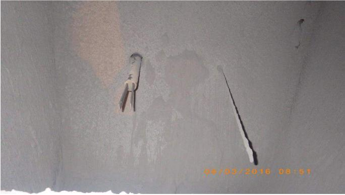
Photo 28 - Baghouse 1 - Hopper Level probe - Installed With Correct Orientation (Gap vertical)
