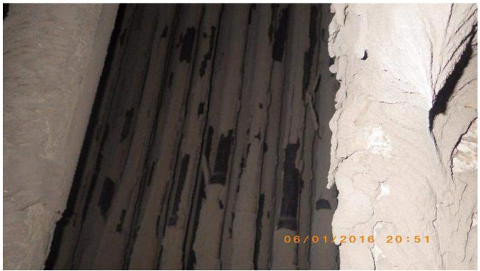
Photo 11 - Upper 3rd Pass – View Looking into Superheater – Screen Tube Fouling Heavy Near Door
