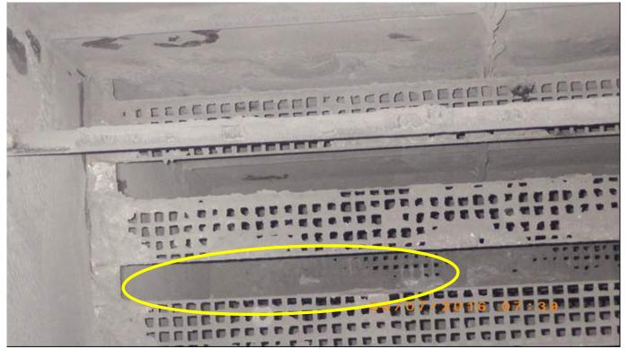
Photo 39 - Close up view of Inlet To Baghouse Inlet Duct – 2<sup>nd</sup> Row of Baffle Screens Remained Partially Plugged (as left)
