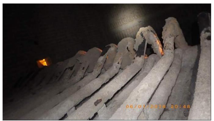
Photo 10 - 3<sup>rd</sup> Pass Convective Zone Bypass Loops – Looking Up
