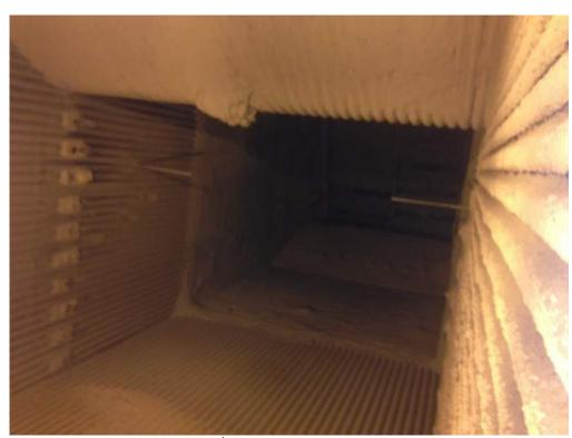
Photo 3 – 1<sup>st</sup> Pass Small Build Up on Bullnose
