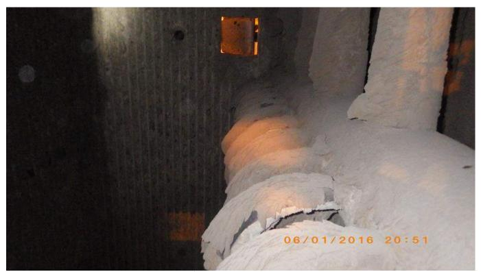
Photo 12 - Top of 3<sup>rd</sup> Pass – Header at Bottom of Screen Tubes
