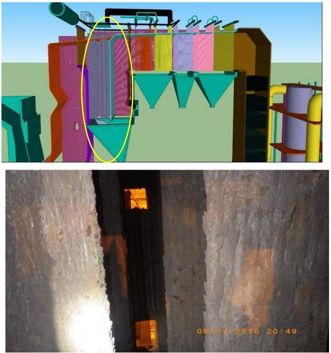
Photo 7 - 2<sup>nd</sup> Pass Superheater Platens.
