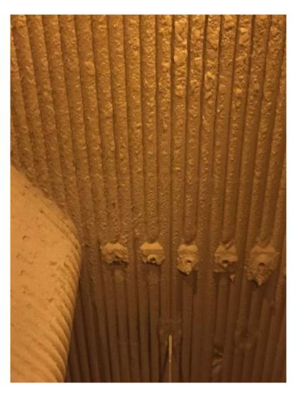
Photo 2 – Boiler 1<sup>st</sup> Pass – IGR Nozzles
