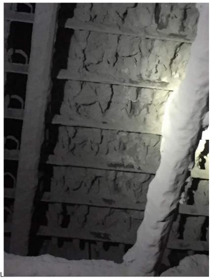
Photo 26 - View up at bottom of Bags – Fouled Build up That Appears to Have Formed When Moist or Wet (NOT TYPICAL)
