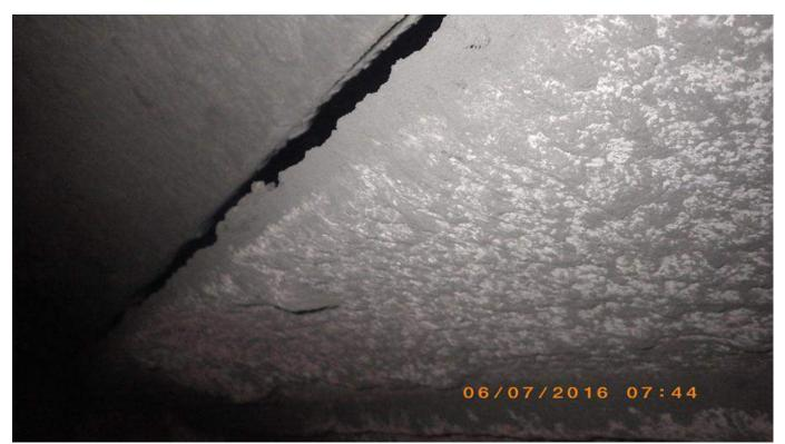
Photo 33 - Damper between Quench and Dry Reactor. Only Slightly Open – Forces air down into Conditioning Rotor
