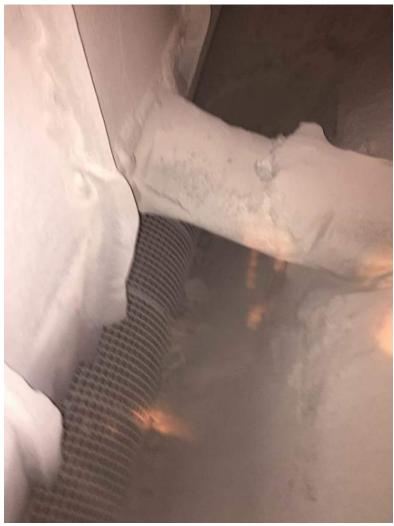
Photo 34 – Lime Screw Feeder (center)– Plugged (as found )
