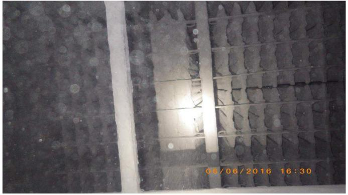
Photo 45 - One Set of Bags in Boiler 2 Cell 2 were Plugged – All Others Clear (Better than Unit 1)
