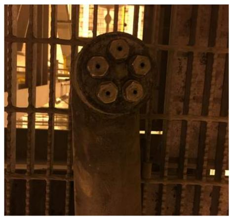
Photo 32 - Spray Nozzle – New Condition
