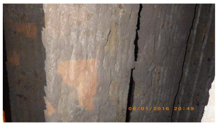
Photo 8 - Second Pass Superheater Platen – Expected Fouling
