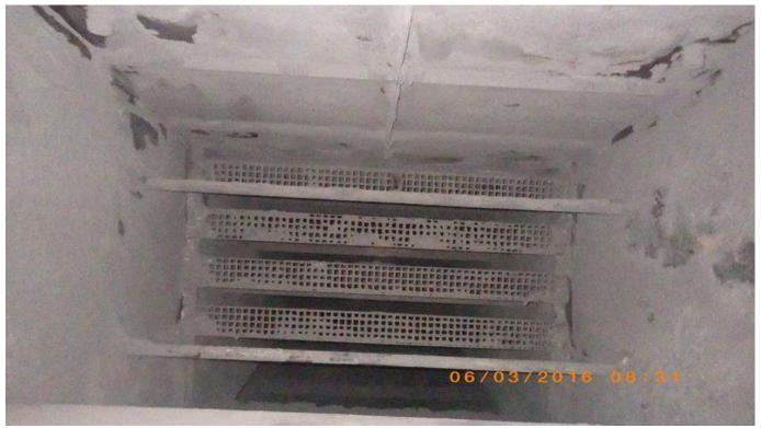
Photo 38 - Inlet To Baghouse Inlet Duct – Baffle Screens at Far End Cleared during Boiler #1 Shutdown (as left)
