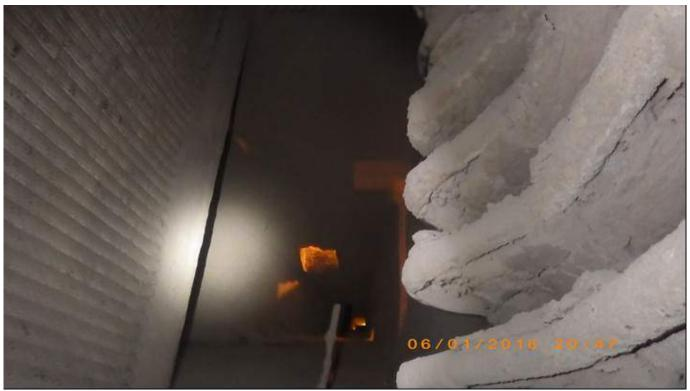
Photo 9 - 3<sup>rd</sup> Pass Rear wall – Loops from Convective Zone Removal on Rear Wall (left side of photo) Hopper Clear (At bottom) No Fouling on Front Wall
