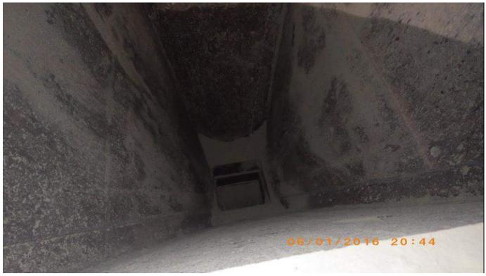
Photo 16 - Hoppers under Superheater Sections - all Clear
