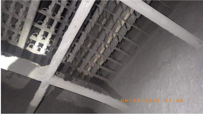
Photo 21 - Bottom of Baghouse Bags – Replaced bags are Evident
