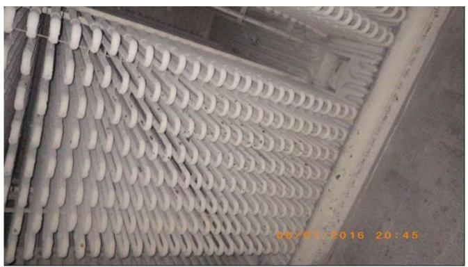
Photo 15 - View Up From Hopper Looking at Superheater Bottom Loops – Fouling Normal to Low
