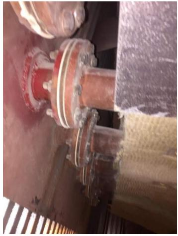
Photo 4 - IGR Nozzles - Boiler Sidewalls
