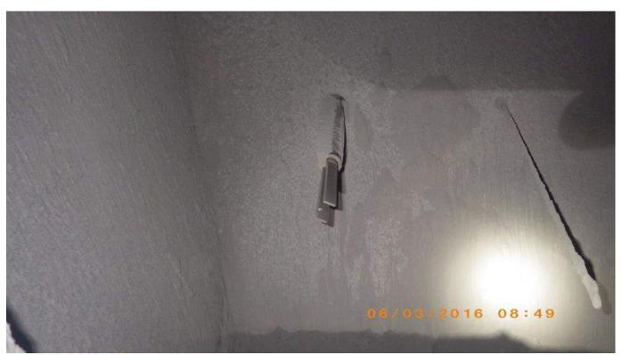
Photo 27 - Baghouse 1 -Hopper Level probe – Installed With Incorrect Orientation (Gap should be vertical)
