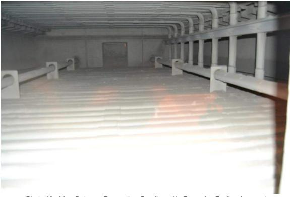
Photo 18 - View Between Economizer Bundles – No Excessive Fouling Apparent
