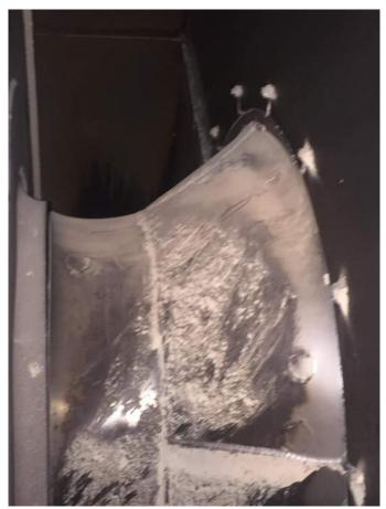
Photo 44 - IGR Fan Inspected – Some Holes in Housing – Refractory lined Inlet Holding up Well
