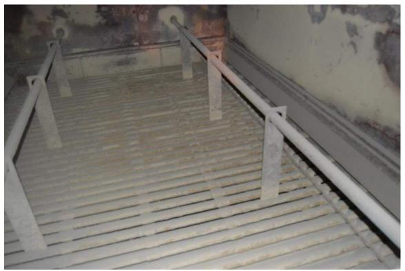
Photo 17 - Inlet to Economizer - No Excessive Fouling Noted from Above
