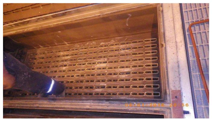
Photo 19 - Baghouse Tube Sheet - Dust Indicates Bags in That Area Have Been Pulled for Replacement or Inspection
