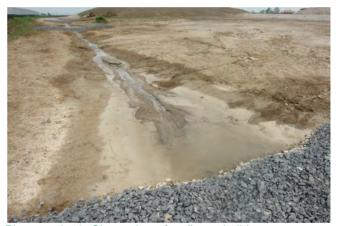
Photograph 10: Closer view of sediment build-up at upstream end of furthest downstream rock-check dam on May 29, 2012
