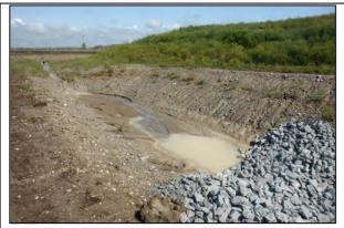
Photograph 31: View looking north at rock check dam within western interceptor swale, along with well vegetated Stock Pile #1 on September 5, 2012
