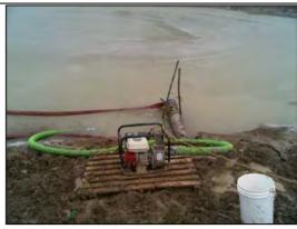
Photograph 56: Closer View of West SWM Pond incl temp PVC outlet pipe, with no controlled discharge, during (prespring) freshet conditions on March 12, 2013
