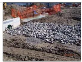
Photograph 70: Closer View of eastern interceptor swale on April 15, 2013
