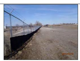
Photograph 66: View of southern perimeter silt fence on April 15, 2013
