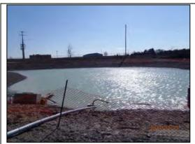
Photograph 67: View of East SWM Pond incl temp PVC outlet pipe on April 15, 2013
