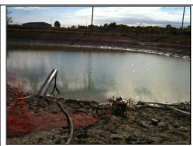
Photograph 43: View of East SWM Pond (incl temp PVC outlet pipe well above water level, with no controlled discharge), during sampling visit on September 28, 2012
