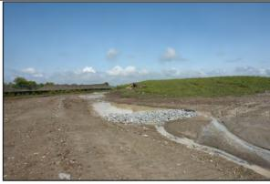
Photograph 32: View looking north and upstream along western interceptor swale and rock check dam in need of repair on September 5, 2012
