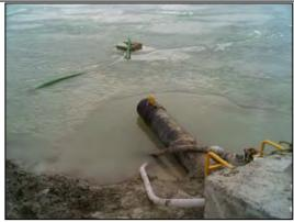
Photograph 55: View of East SWM Pond incl temp PVC outlet pipe, with no controlled discharge, during (pre-spring) freshet conditions on March 12, 2013
