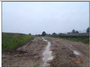
Photograph 19: View looking south capturing Stock Pile #1, western perimeter swale and silt fence on June 12, 2012
