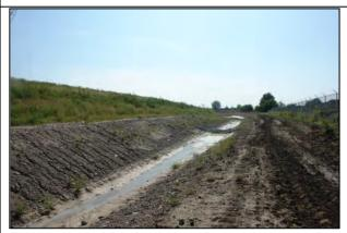
Photograph 33: View looking south capturing western perimeter silt fence and interceptor swale on September 5, 2012
