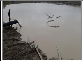
Photograph 26: Closer View of W-SWMP-OUT location showing outlet invert versus water level on June 28, 2013
