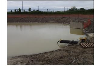
Photograph 25: Closer View of E-SWMP-OUT location showing outlet invert versus water level on June 28, 2013
