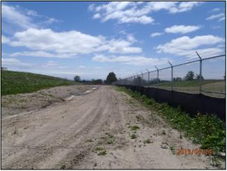
Photograph 1: View looking south capturing Stock Pile #1, western perimeter swale and silt fence on May 24, 2013
