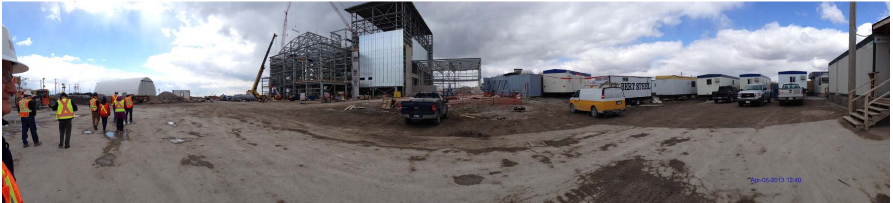
Photo 1: Looking west from inside inner security site access gate
