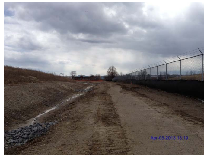
Photo 20: Looking south showing erosion control measures in west drainage ditch
