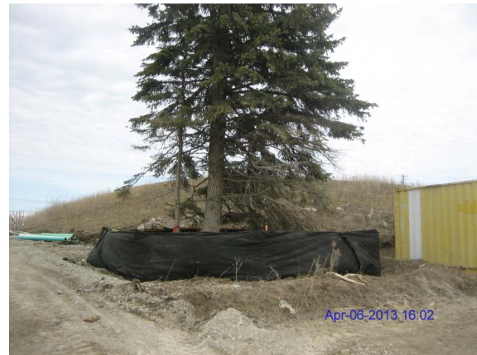
Photo 10: : Norway Spruce enclosure as reported by Region of Durham staff on 13/04/09
