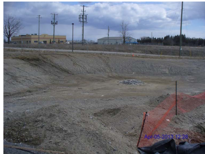
Photo 14: Looking southeast at southeast storm water management pond
