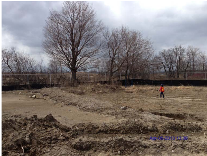
Photo 17: Looking southwest showing monitoring wells perimeter fence with silt curtain and sugar maple across fence
