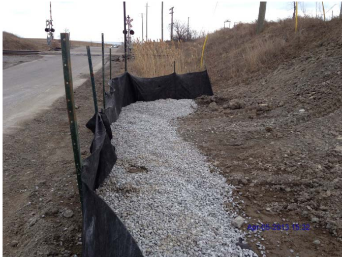
Photo 15: Looking south at east side of perimeter fencing at the southeast corner showing silt curtain installed
