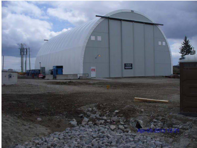
Photo 7: Looking southeast showing temporary construction facility
