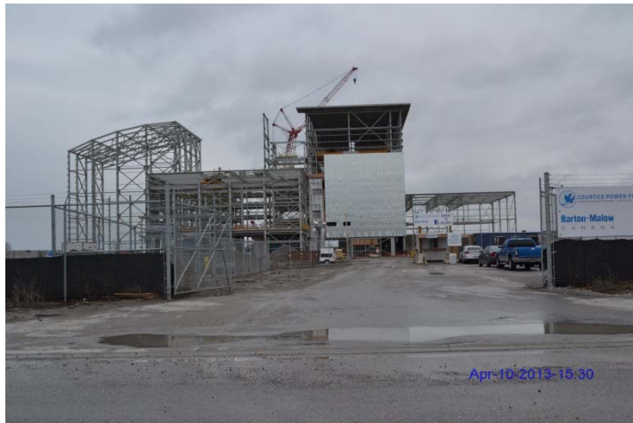
Photo 5: View of controlled site access gate and inner security gate
