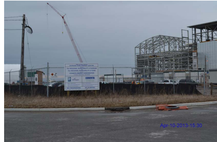
Photo 4: Site entrance sign
