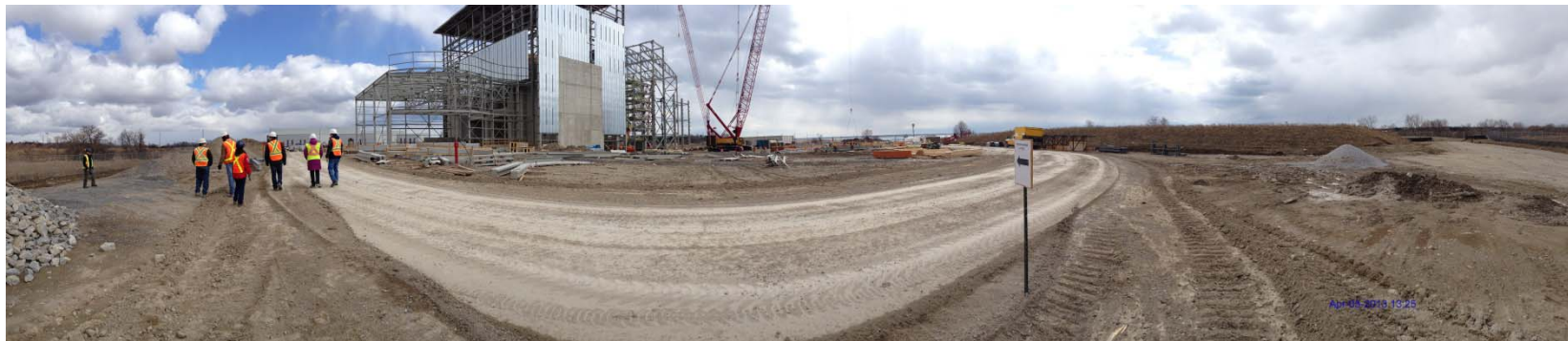
Photo 22: Looking southeast from northwest corner of site
