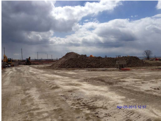
Photo 11: Looking south showing temporary soil stockpiles
