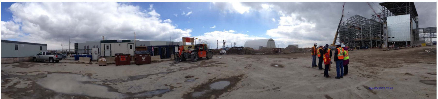
Photo 2: Looking south from inside inner security site access gate
