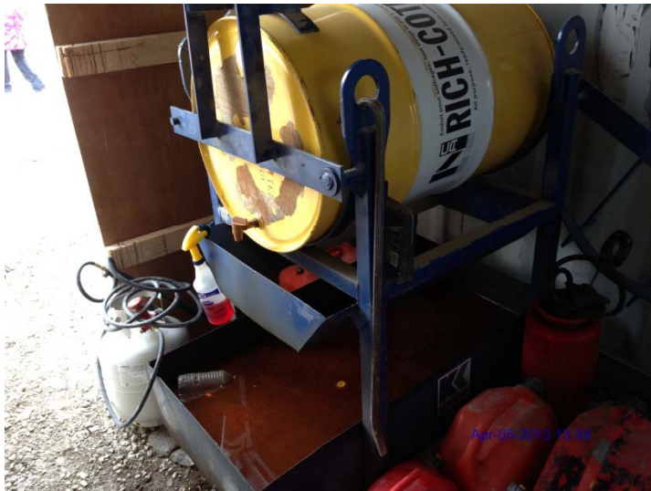
Photo 27: Liquid fuels tank with secondary containment
