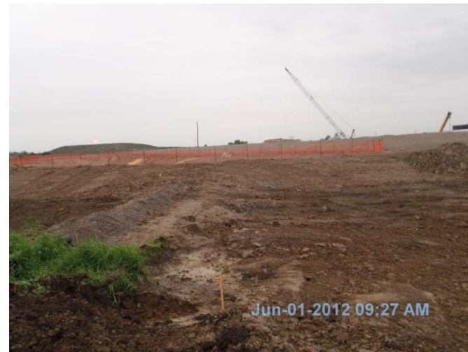
Photo 16: Looking north across site from southwest corner.
