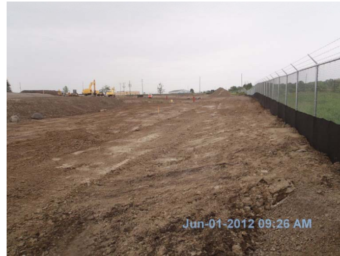
Photo 14: Looking east along south property line.
