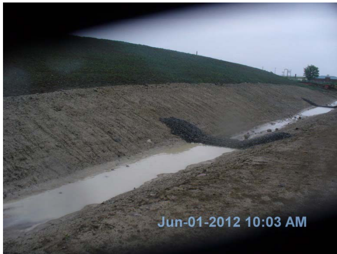
Photo 26: Drainage swale along west fence line with check dams present - seeded soil storage pile in the background.
