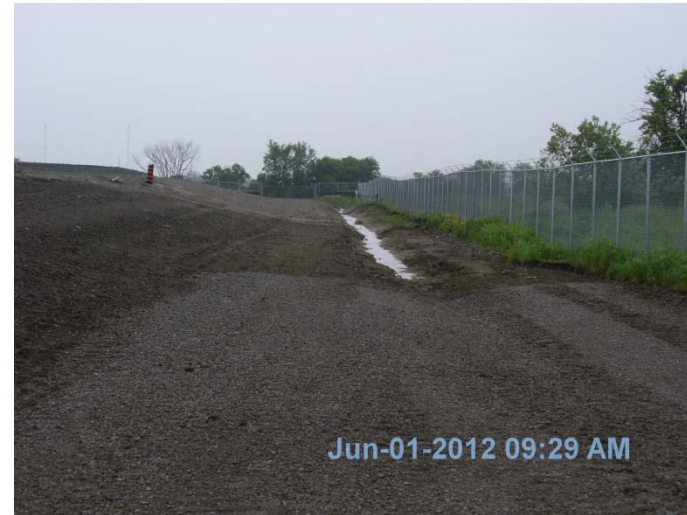
Photo 29: Drainage swale along the property line looking west.
