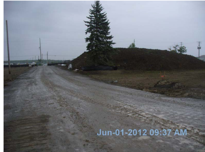
Photo 2: Protected tree (spruce) with surrounding fabric barrier - raised gravel access road to east fence line and site exit.
