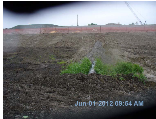
Photo 18: looking north to the west storm water management pond discharge pipe visible in foreground.
