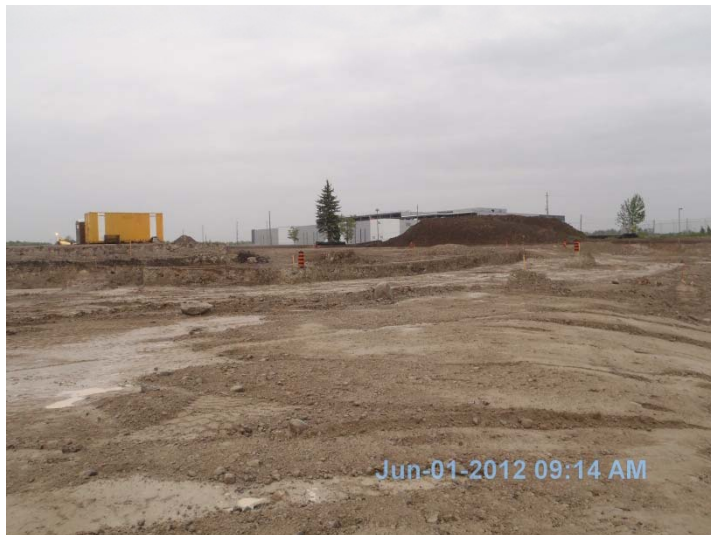
Photo 7: Looking northeast along east property line from southeast corner of site.
