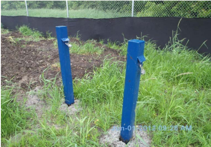
Photo 13: Monitoring wells installed at southwest corner of the site.
