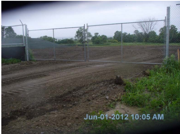
Photo 28: View of locked access gate at northwest corner of site.
