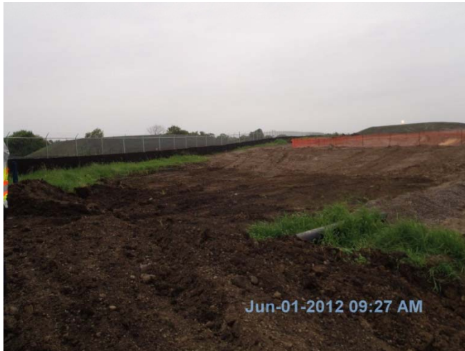
Photo 17: Looking northwest across the site from the southwest corner.
