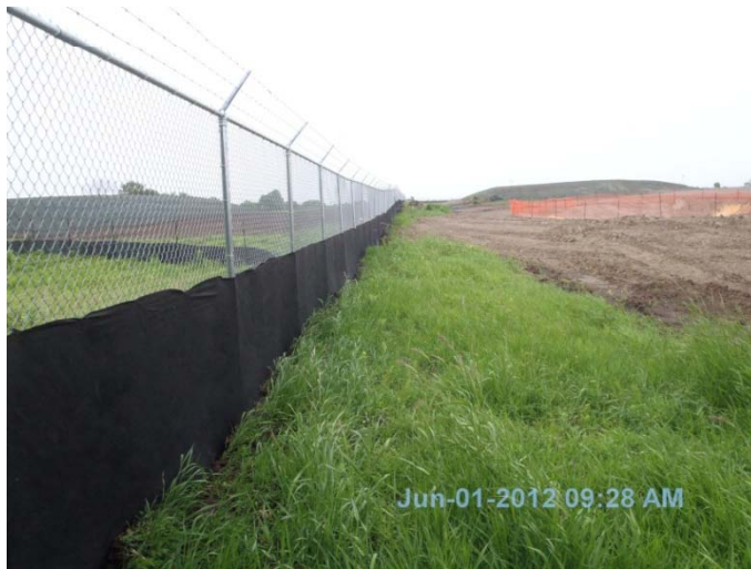
Photo 21: Looking north along west property Line, showing sediment control.
