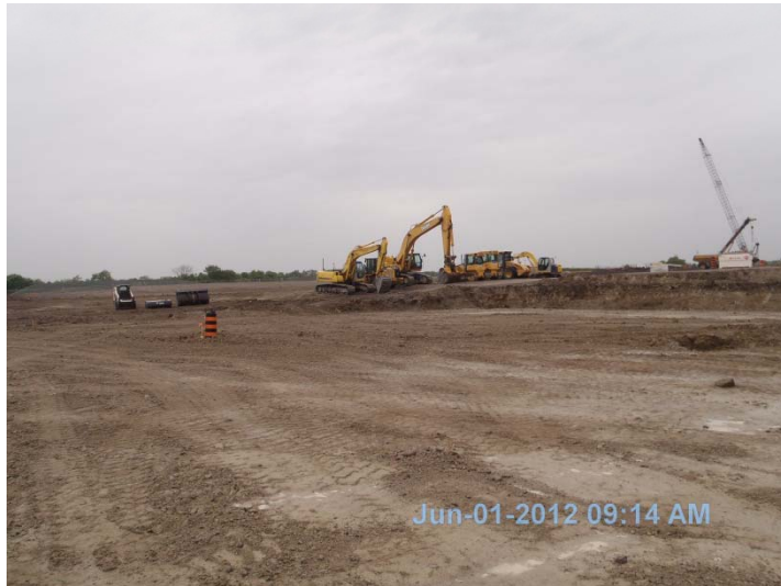
Photo 5: Looking northwest across site from southeast corner of site.
