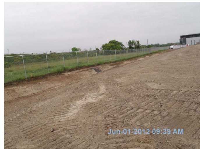
Photo 31: View of north fence line and drainage swale looking northeast.
