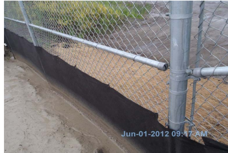
Photo 10: Silt curtain and erosion control carpet at southeast corner.
