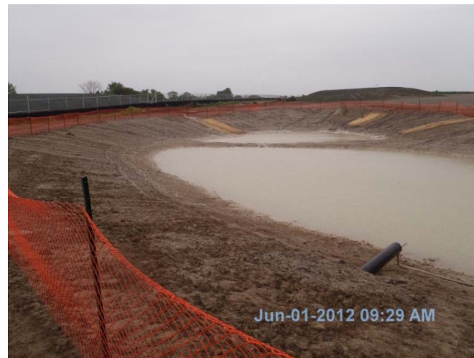
Photo 24: Looking northwest at west storm water management pond.
