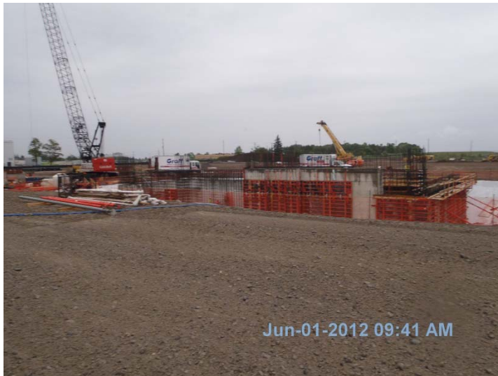
Photo 32: View of building construction progress, view from north looking south.
