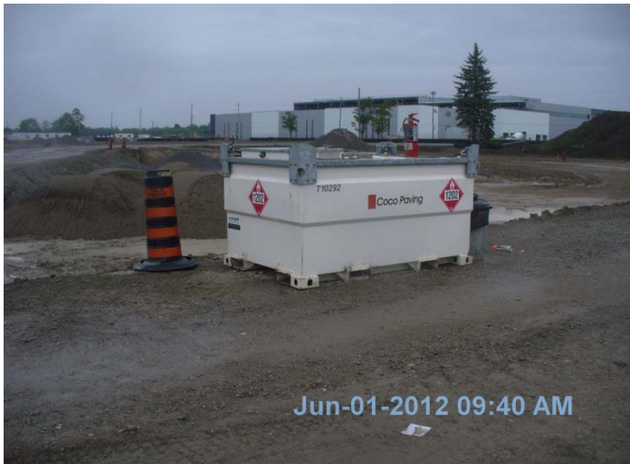
Photo 3: On-site fueling depot with secondary containment for stored fuel, fire extinguisher and placards present.
