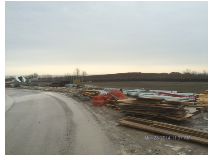
Photo 10: Looking southwest at west portion of site.
