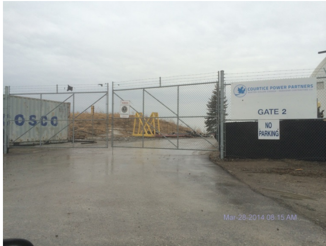
Photo 5: Exterior view of controlled entrance.
