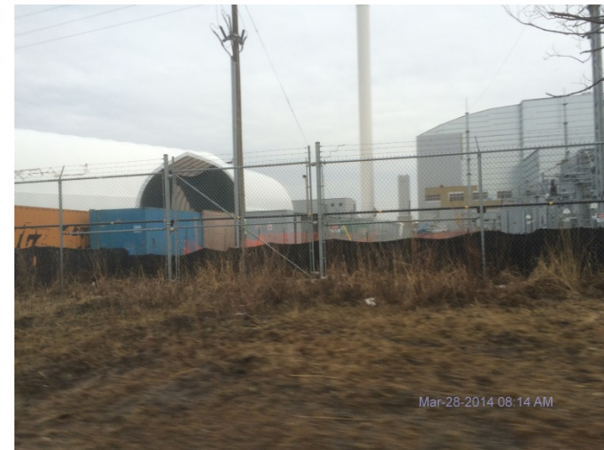
Photo 4: Exterior perimeter view of fencing and silt curtain
