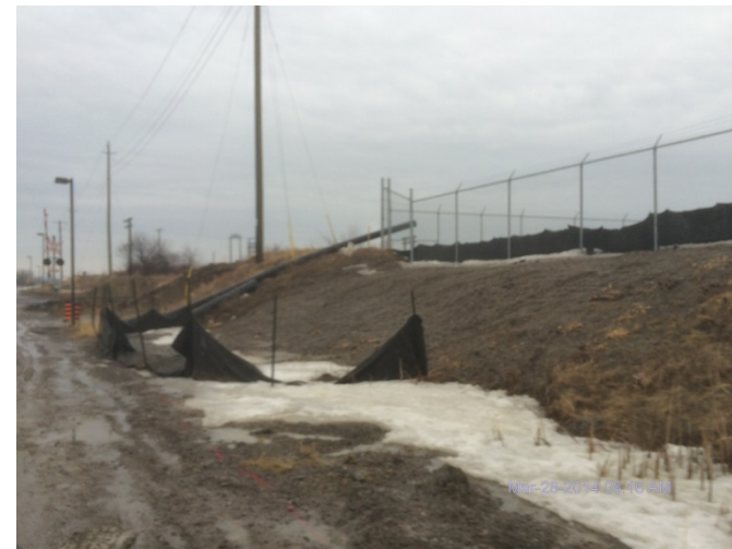
Photo 28: Silt curtain outside of southeast corner at commencement of audit
