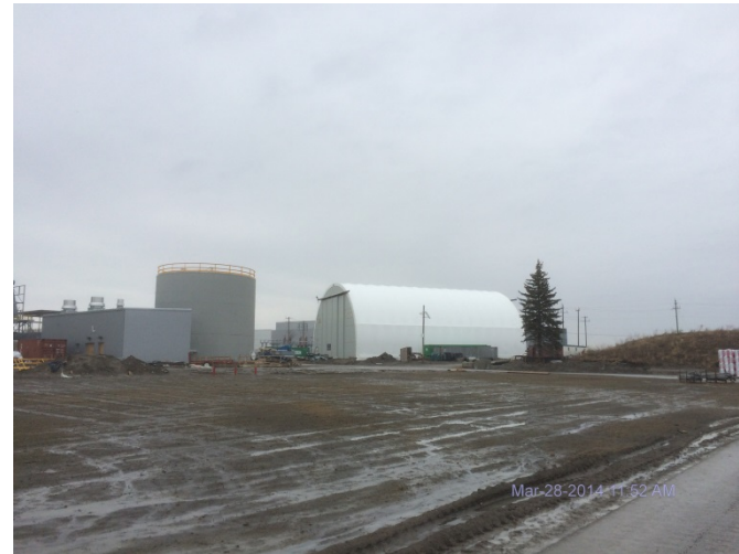
Photo 20: Looking north showing site grading.
