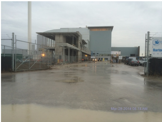
Photo 3: Showing controlled main entrance to site.
