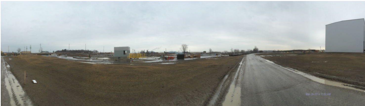
Photo 21: Panoramic looking along south of the site.
