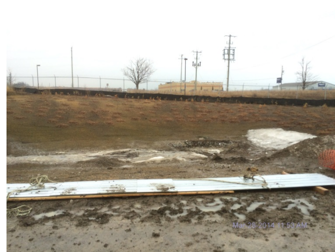
Photo 24: looking east at drainage to southeast corner stormwater management pond.
