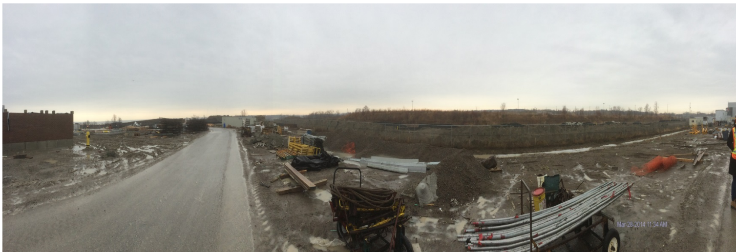
Photo 11: Panoramic view along north of site showing construction materials laydown area.
