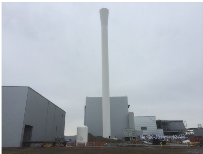
Photo 23: Looking north showing status of site construction.
