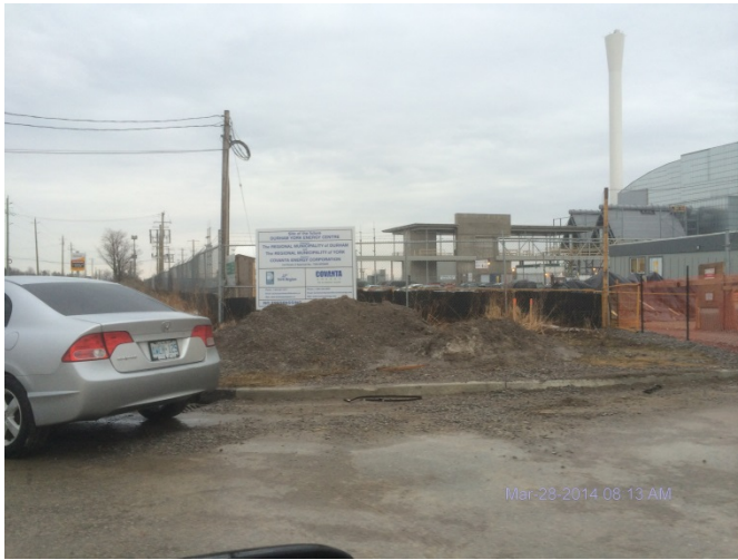
Photo 1: Project sign at northeast corner of site.
