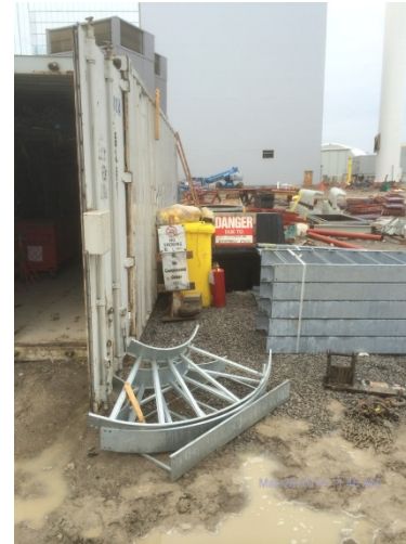
Photo 16: Liquid fuel storage west of main building.
