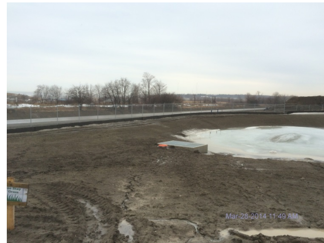
Photo 18: Stormwater management pond at south west corner of site.
