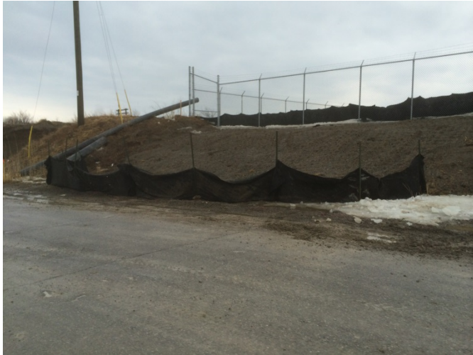
Photo 29: Silt curtain outside southeast corner fence at completion of audit.
