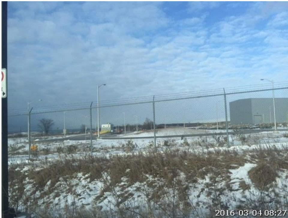
Photo # 02 looking west from Osborne Road to weigh scales, showing site perimeter fencing
