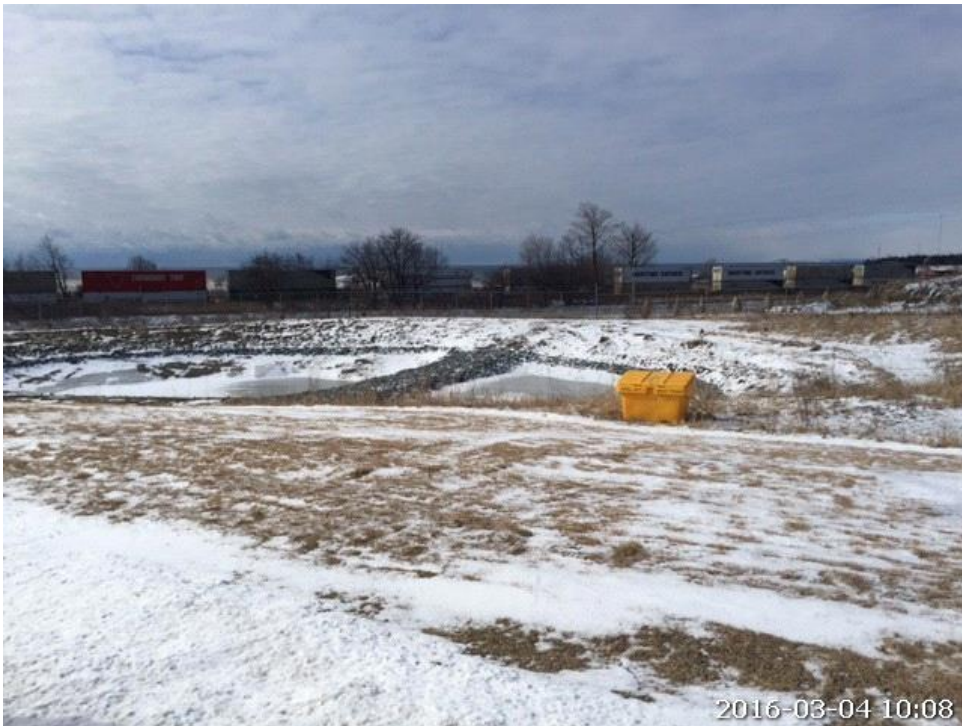
Photo # 10 looking southwest towards stormwater management pond with spill response kit in foreground
