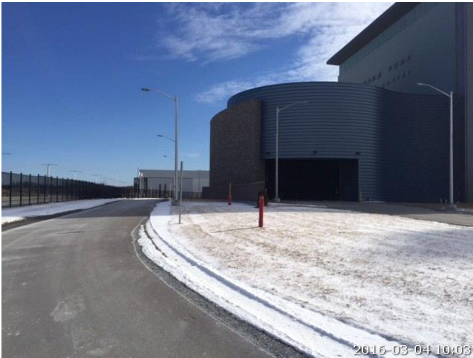
Photo # 08 looking east along the internal access road along the north of the facility
