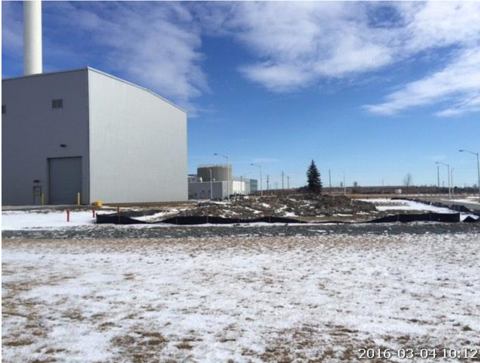
Photo # 11 looking east showing stockpiled soils from stormwater management cleanout
