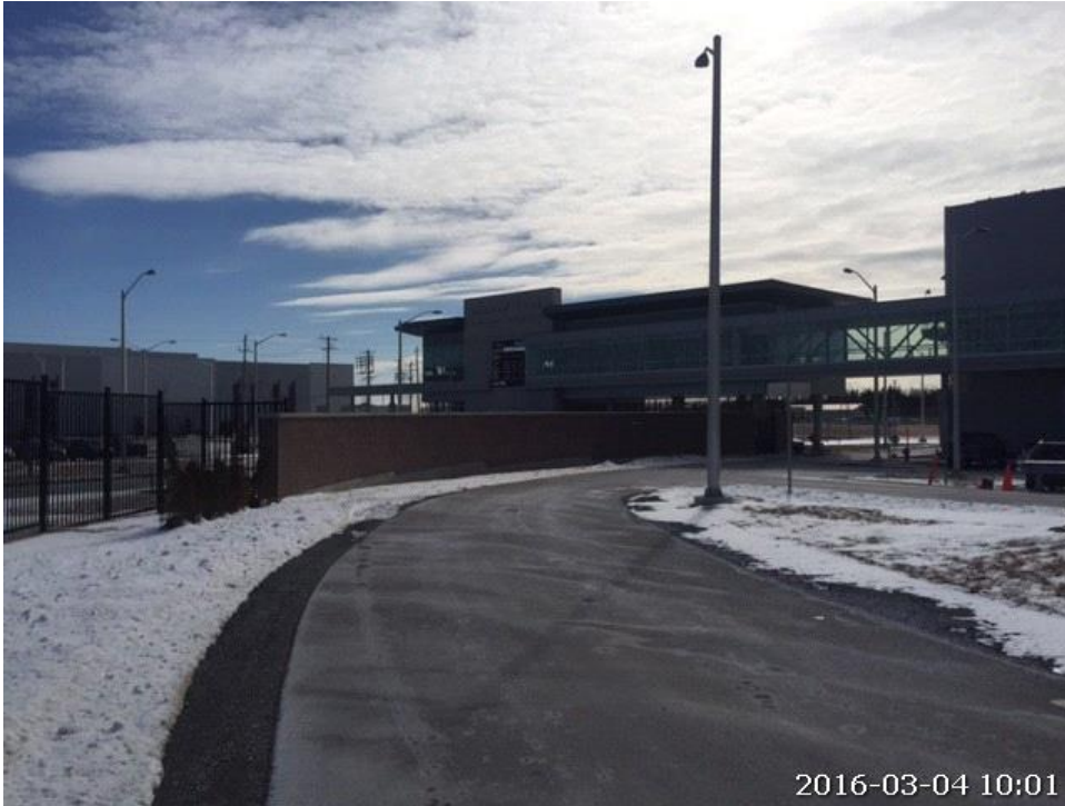
Photo # 07 looking southeast along internal access road towards visitor center
