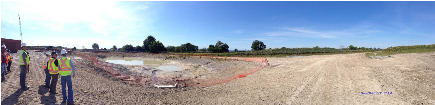
Photo 3: Panorama view from south to northwest in the southwest corner
