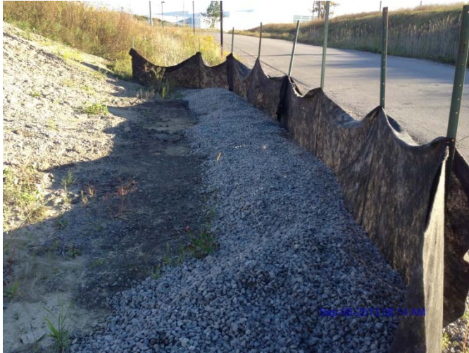
Photo 29: Showing stone on silt curtain at regraded southeast corner entrance
