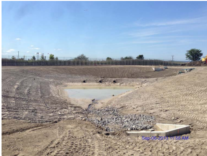
Photo 21: Looking south across east storm water management pond
