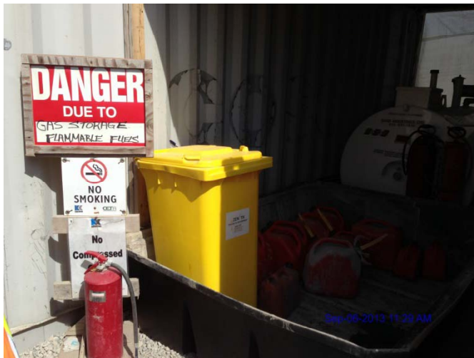
Photo 7: View of entrance to liquid fuels area
