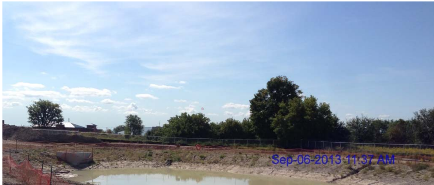
Photo 13: Looking southwest showing west storm water management pond in the foreground
