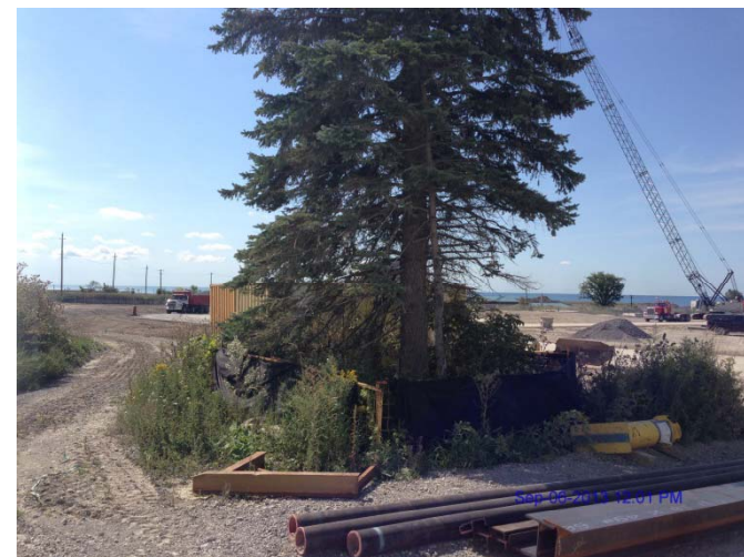
Photo 24: looking southwest at the spruce tree showing fencing and silt curtain
