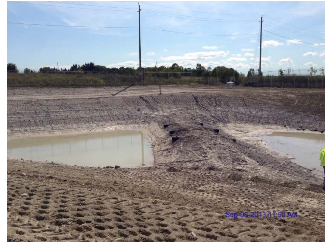
Photo 18: Looking southeast at east storm water management pond
