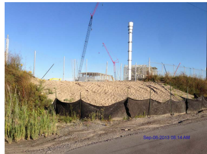
Photo 28: Southeast corner entrance that had been regraded showing silt curtain
