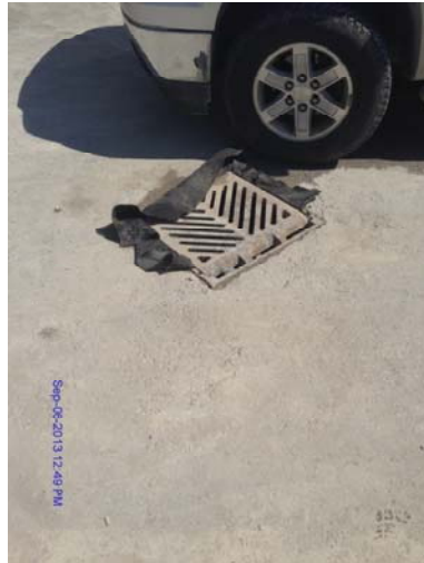
Photo 25: Catch basin in parking lot with silt curtain barrier
