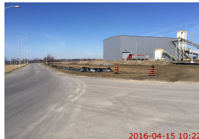
Photo 8: looking northwest showing stockpiled soils from west corner storm water management pond cleanout. To be removed from site when half load restrictions come off roads.
