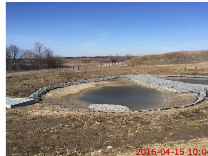
Photo 4: looking west across west storm water management pond, with monitoring wells across pond.
