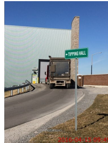
Photo 26: trucks entering the tipping building – doors closed prior to entry..
