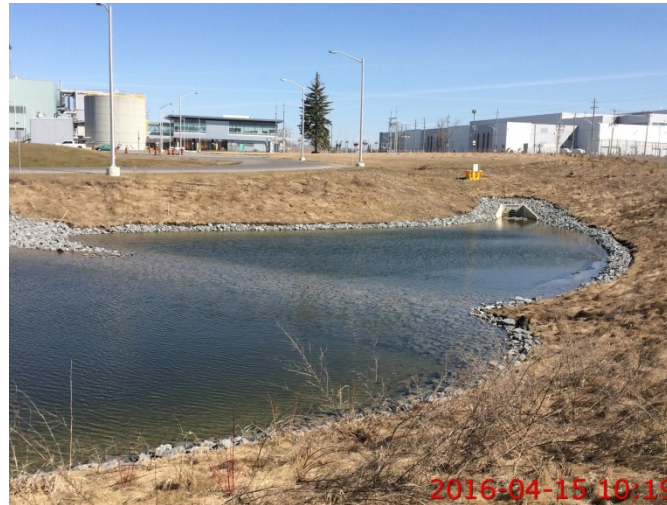
Photo 34: looking north across east storm water management pond.
