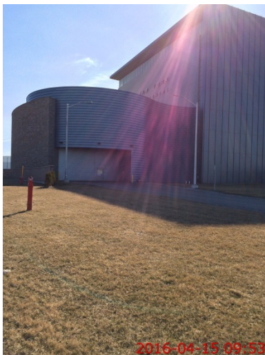
Photo 15: tipping building exit – doors closed when not being used for building egress.
