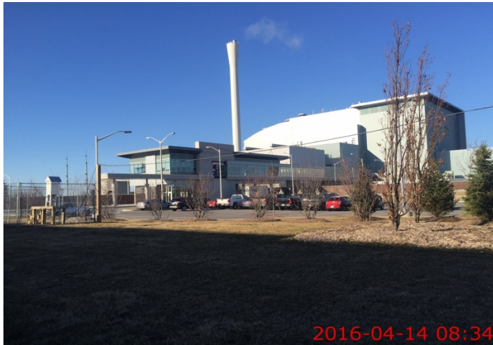
Photo 13: looking southwest across visitor centre parking lot.
