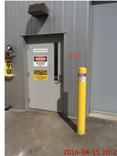
Photo 18: signage on building access.
