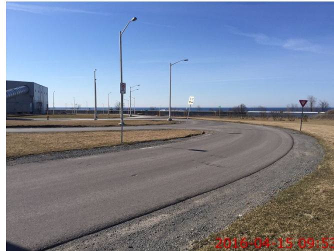
Photo 2: looking south along roadways on west side of facility.
