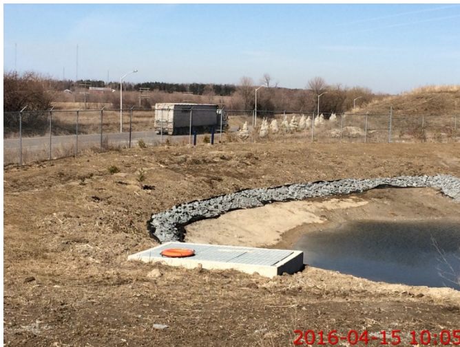
Photo 31: looking southwest across west storm water management pond. Groundwater monitoring wells, landscaping plantings and access road in the background.
