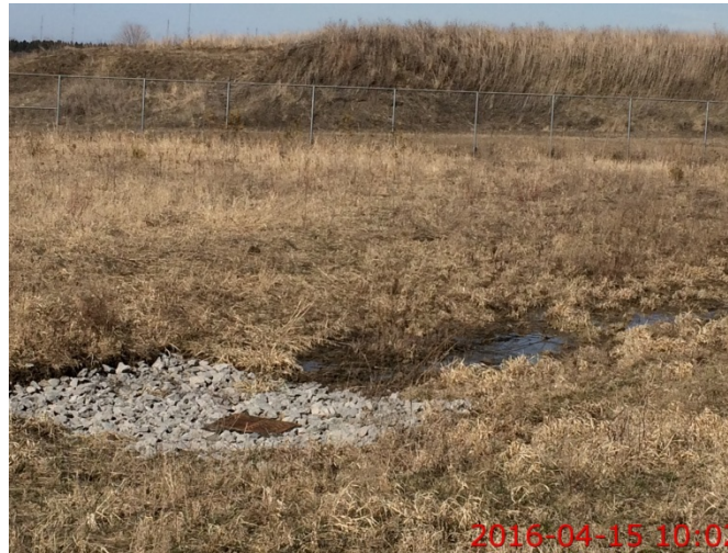
Photo 30: vegetated swale with rock check and catch basin leading to storm water management pond.
