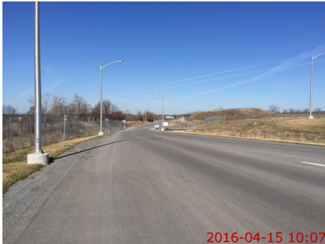
Photo 5: looking west, through gate at fence along the waste receiving road.
