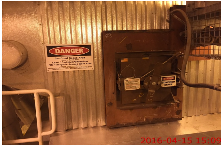
Photo 22: signage on access to furnace.
