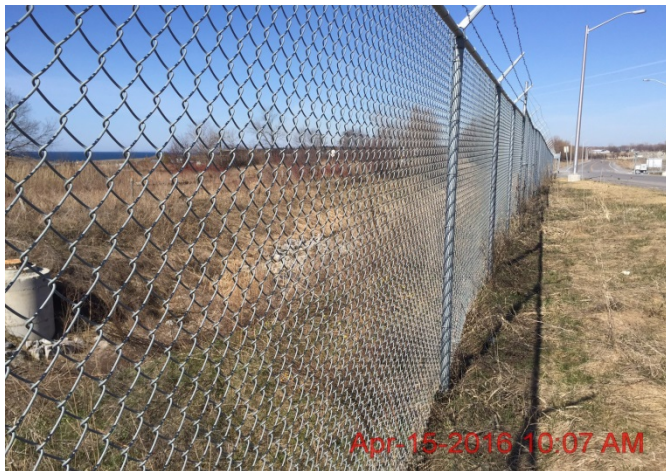
Photo 7: looking west along fencing south of the storm water management pond.
