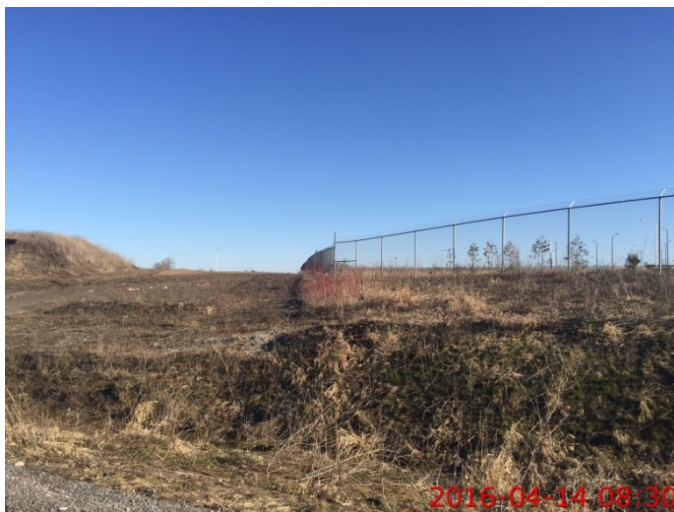
Photo 11: west perimeter fencing, looking north from southwest corner.
